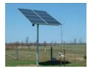
PV modules are designed to be installed outdoors without additional protection. A mounting structure must be constructed to support the modules in all weather conditions.
