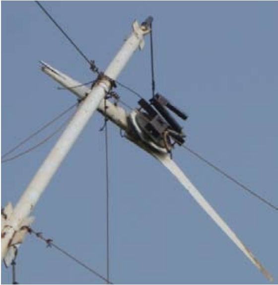
Fig. 42: Tight terminal block avoiding to fall down
