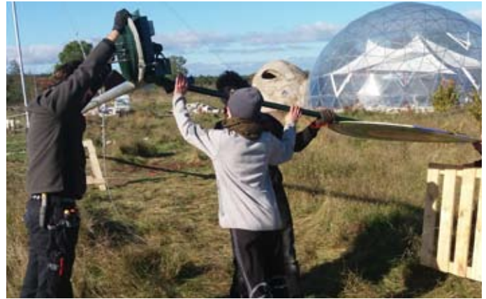
Fig. 20: Installing the tail
