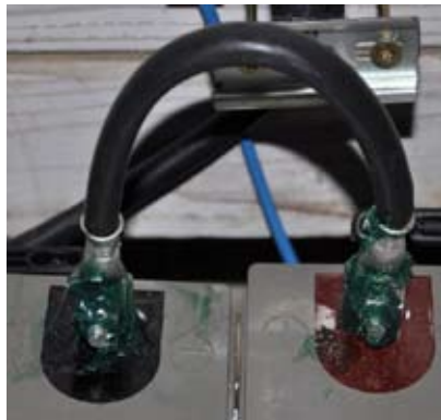
Fig. 55: Grease on connectors
