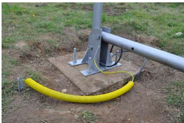
Fig. 2: Ground connection of the tower and electronics
