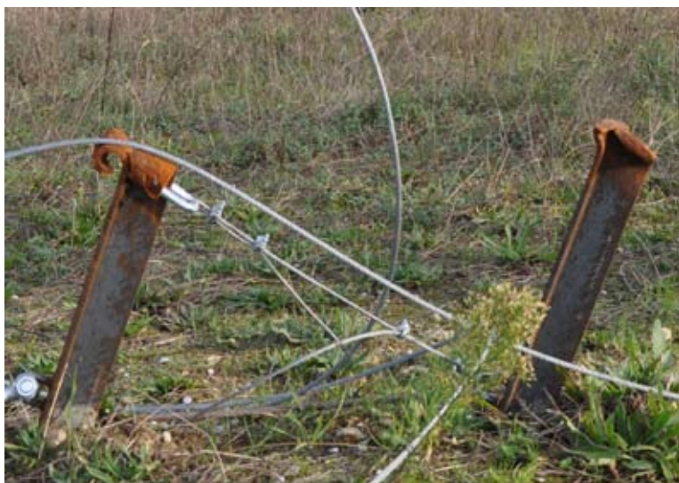
Fig. 49: Secured anchor
