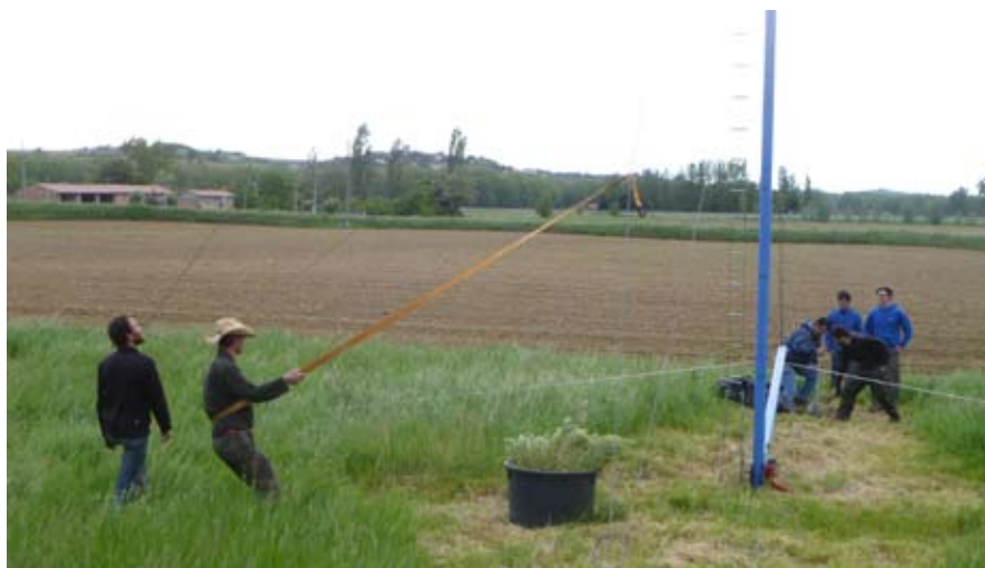
Fig. 14: Pulling top guy wire strap
