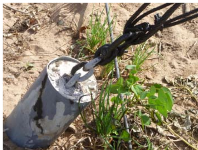
Fig 5 : Chain poured into concrete
