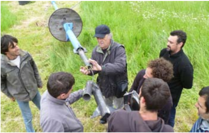
Fig. 19: Installing the alternator & frame
