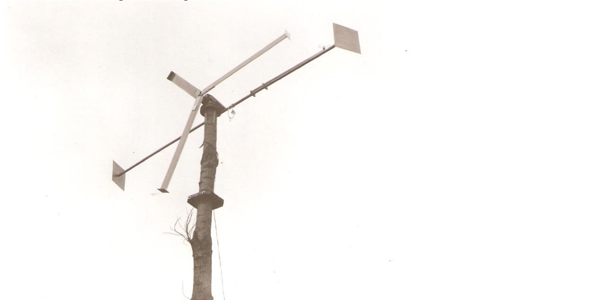
fig. 16 DRIEKA-4 windmill with double vane and tree tower designed in about 1985
